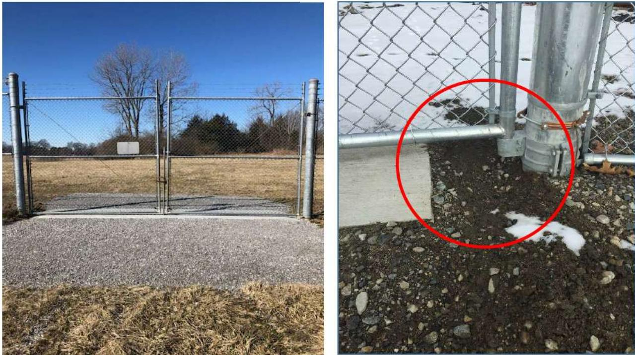
Figure 54. Example of a concrete pad under entrance gate as a wildlife dig-under deterrent. Gap remains large enough for wildlife entrance pictured to the right.
